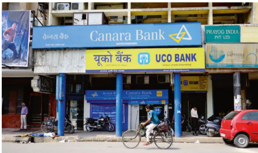
Pillars to be reinforced
